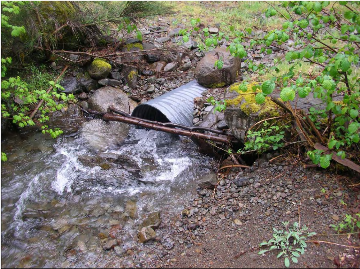
Photo 37. Upstream end of culvert.
