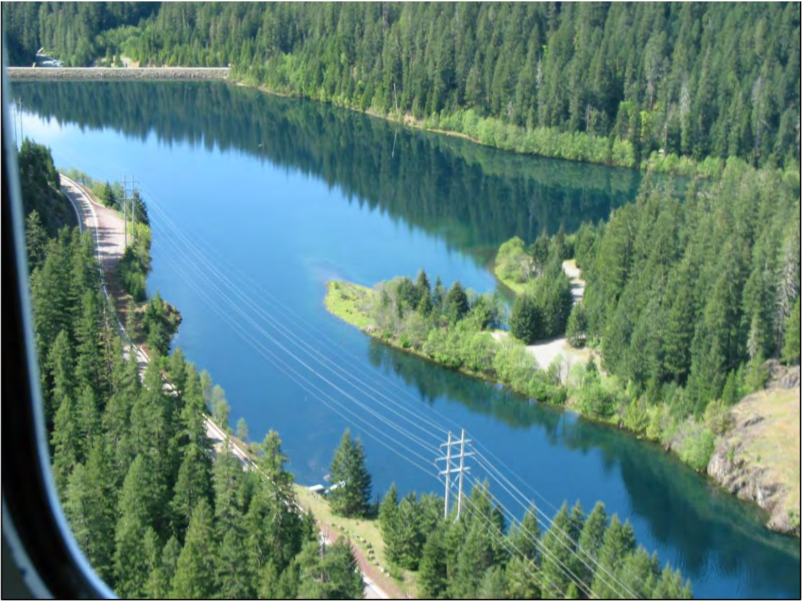
Photo 25. Trail Bridge Dam and Reservoir.
