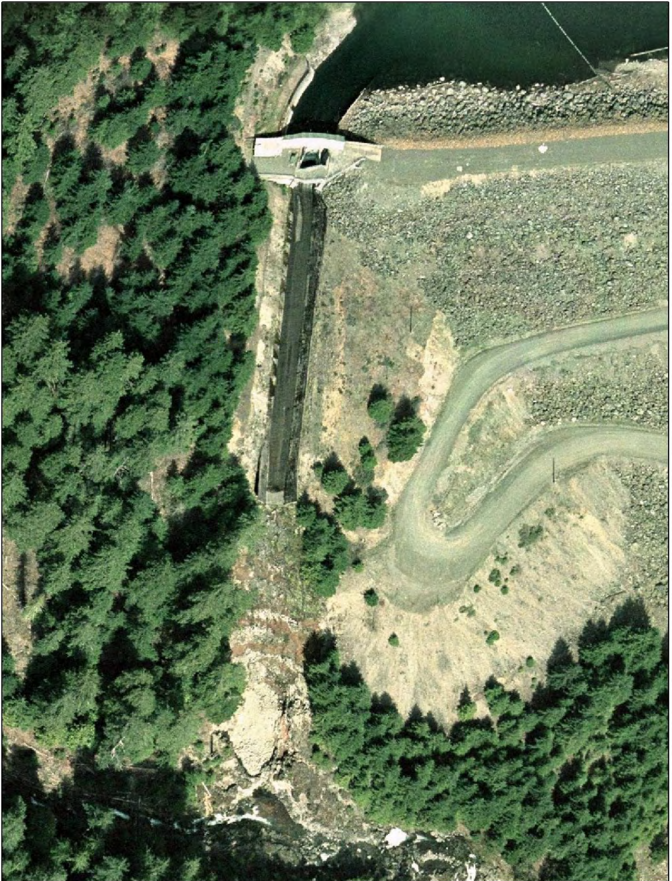
Photo 1. Smith Dam and Spillway.
