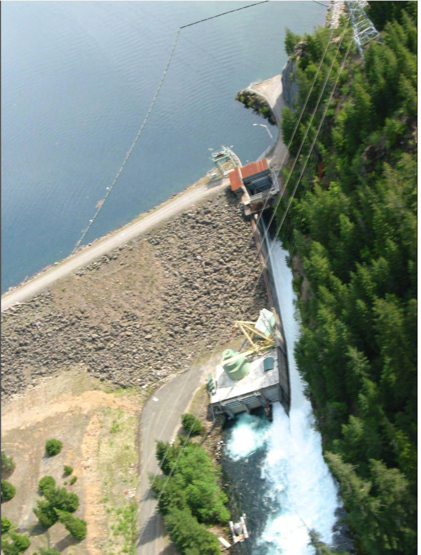
Photo 4. Trail Bridge Dam, Powerhouse, and spillway.
