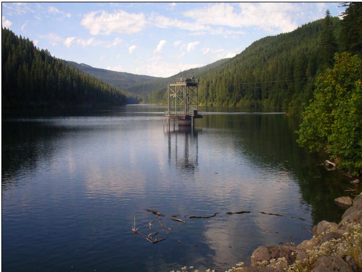
Photo 3. Smith Reservoir and Intake.
