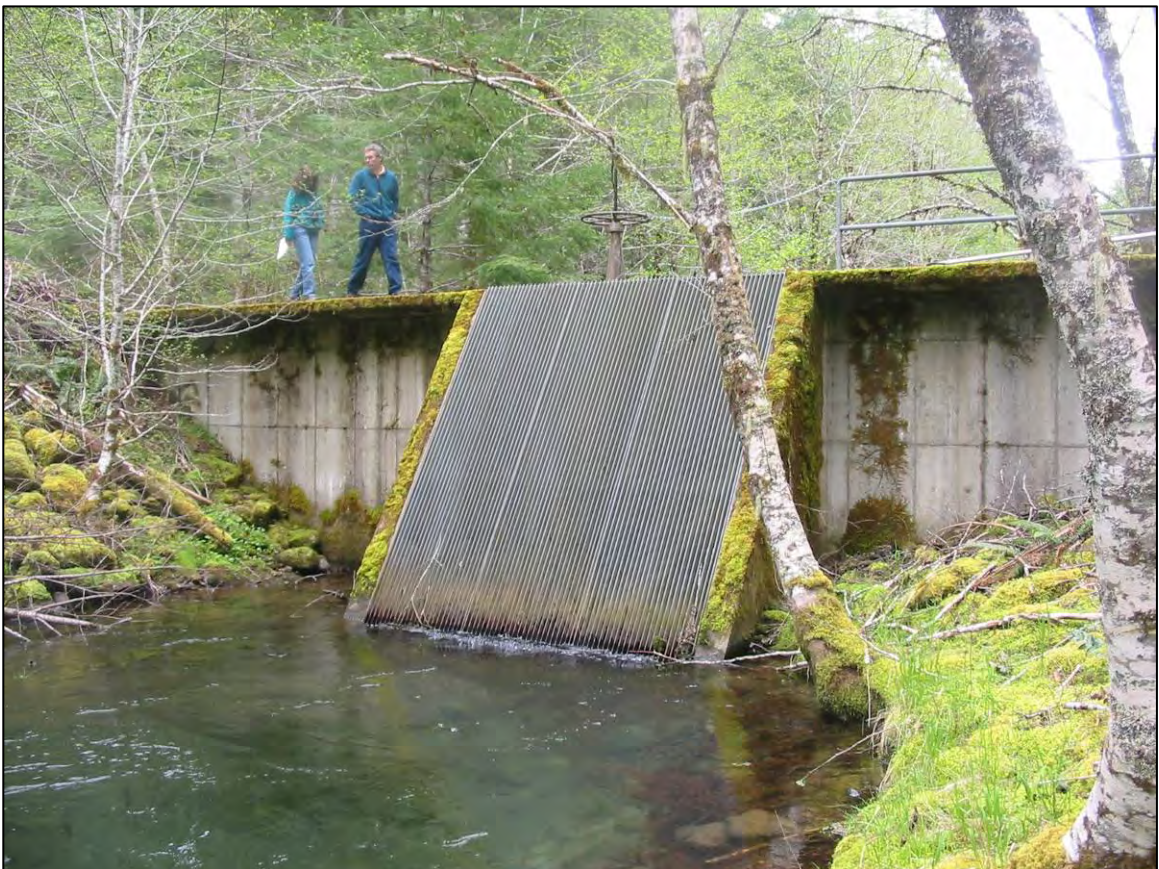
Photo 34. Trash rack at upstream end of the Carmen-Smith Spawning Channel.
