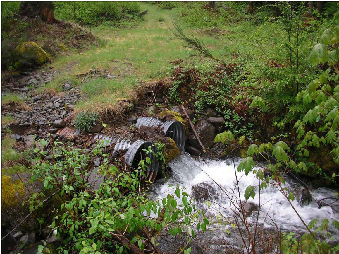
Photo 36. Downstream end of culvert.
