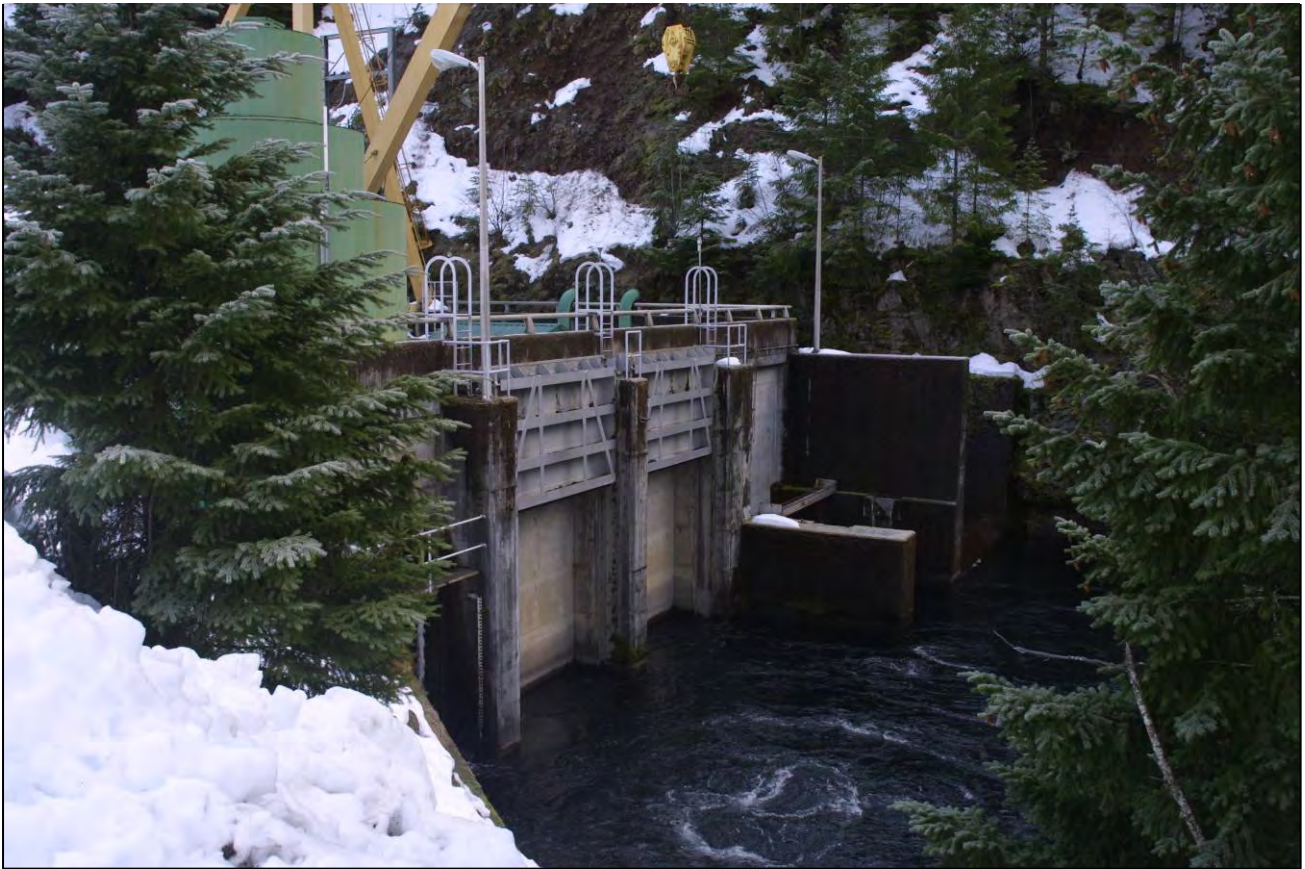
Photo 5. Trail Bridge Powerhouse and spillway, looking upstream.
